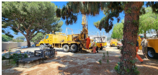
Hollow Stem Auger Drilling at RS- Rinaldi
