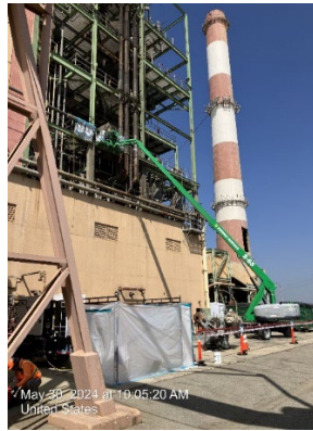
Asbestos abatement 3-stage shower installation.
