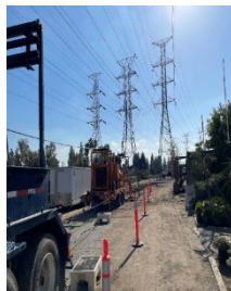
Tower 241: Reconductoring of the Middle Phase
